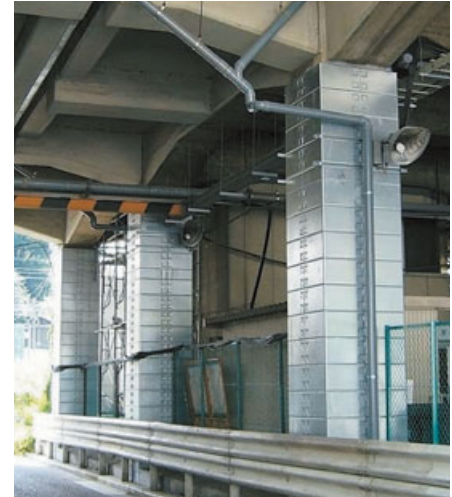
▲Steel Panel Assembly Reinforcement Method
