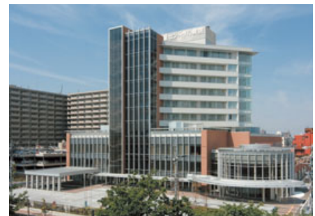
▲Nagoya Central Hospital
