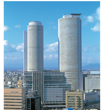
December 20, 1999 Construction of JR Central Towers is completed
