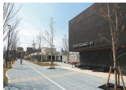
▲NAGOYA CENTRALGARDEN Commercial Complex
