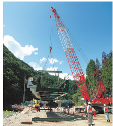
▲Takayama Line's Restoration Work
