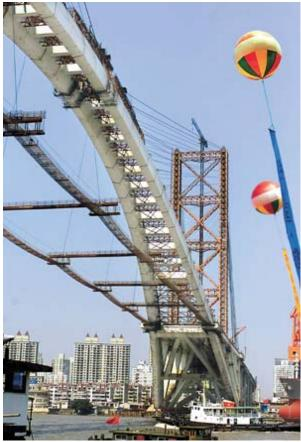
Figure 12: Horizontal cable installation. Ref [9]
