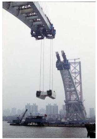
Figure 10: Lifting the arch sections into position Ref. [6]
