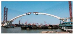
Figure 9: Cable-Stayed Cantilever Construction. Ref. [2]
