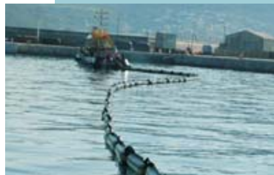
The floating barrier is very effective in containing any possible oil spill.
