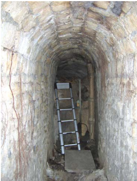
21. Tunnel looking north the reservoir entrance
