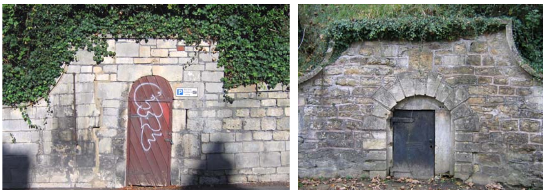
17. The reservoir entrance below Somerset Place (left) and at Cranwells (right)
