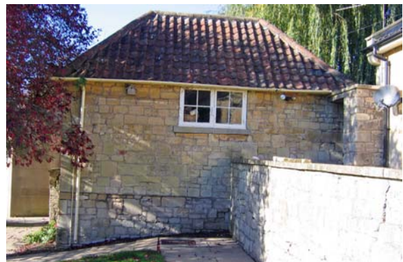
15. Converted garage at rear of no 9 Somerset Place (BRO: BC/626)
