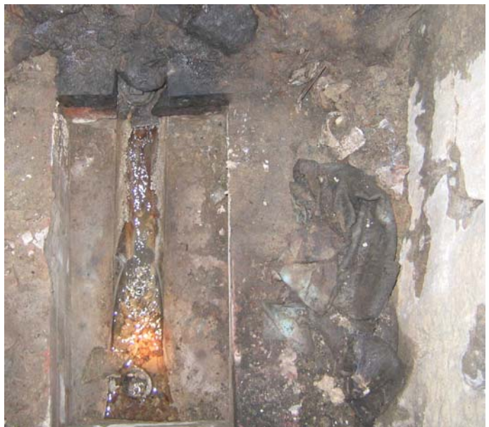
22. drainage pipe below tunnel floor
