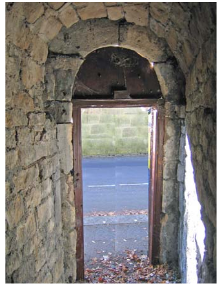
20. tunnel looking south
