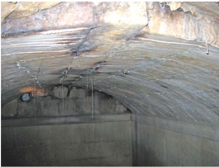
19. Reservoir roof with keystone
