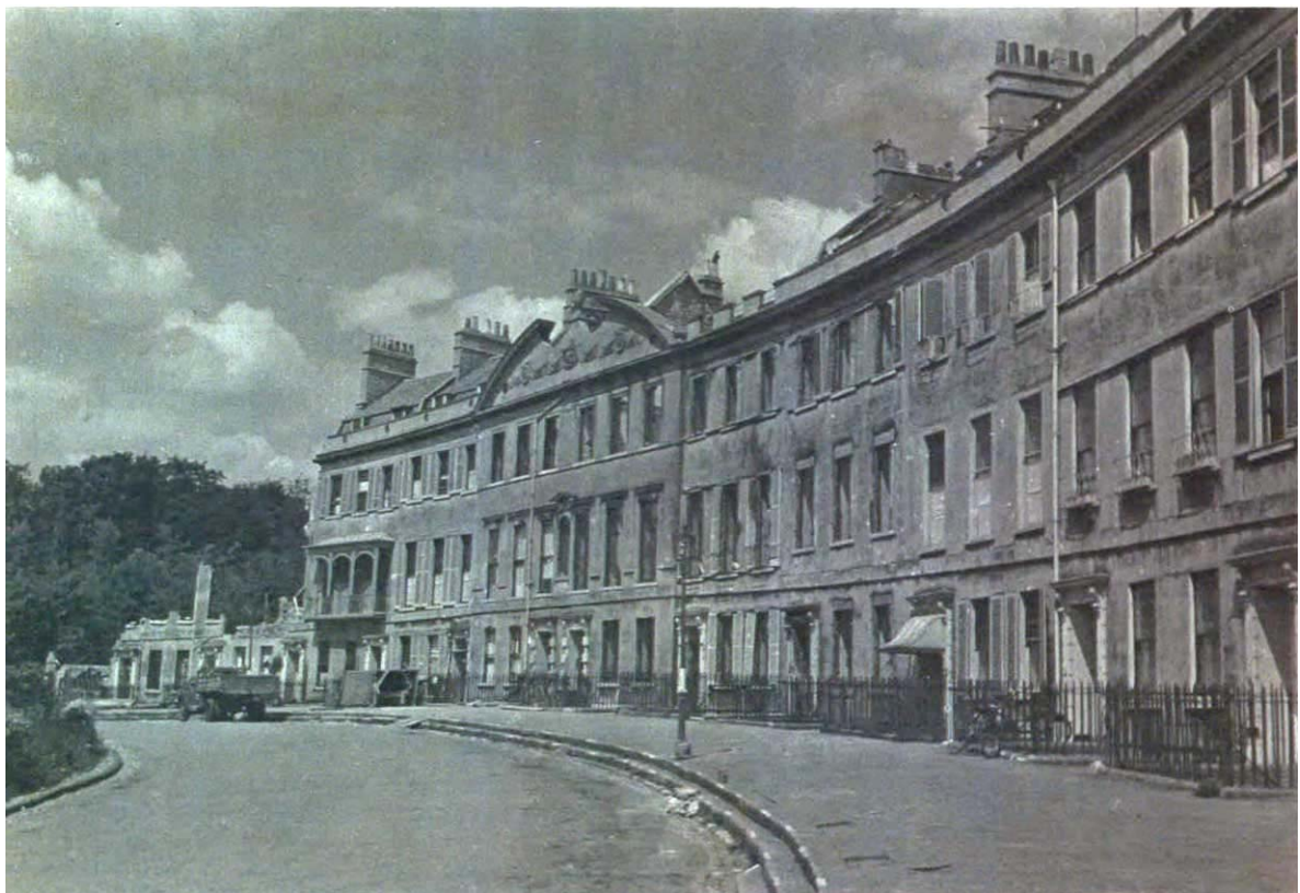
39. 1942 The ruins of 5-7 sp and the remaining façade of nos. 10-11 (BRO: 027)
