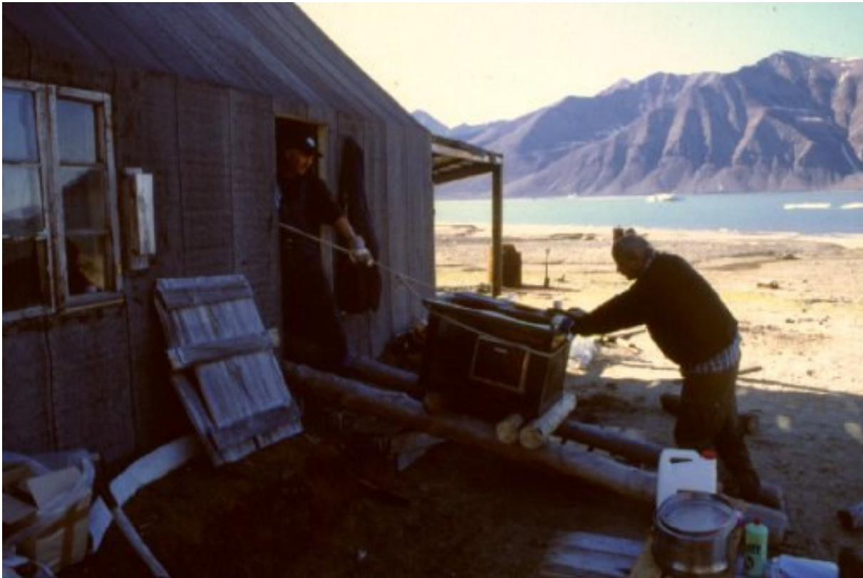
The new stove, weighing 250 kg, is rolled in.
