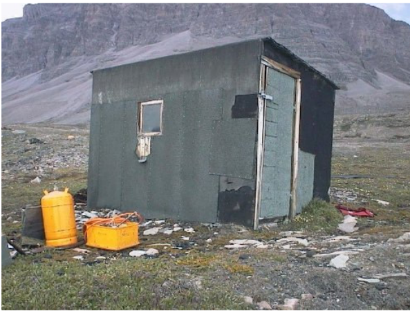
"Kongeborgen" (King's Castle) was inspected and renovated with new felt. Door and window were repaired.
