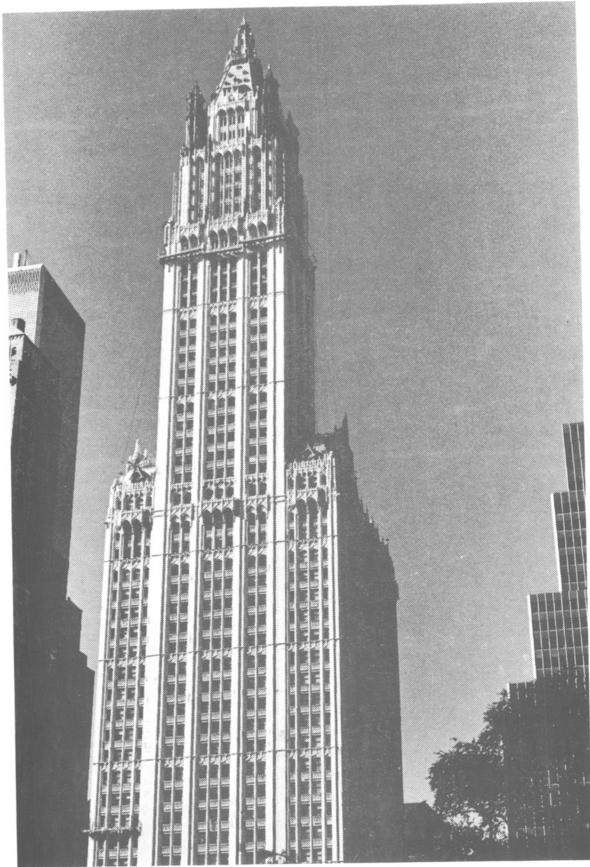
Woolworth Building 233 Broadway Manhattan
