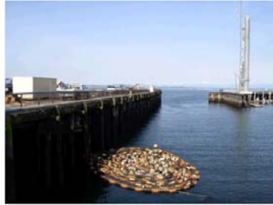
2. View from sidewalk at Pier 62/63 Toward W
