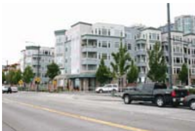
Waterfront Landings Condominiums
