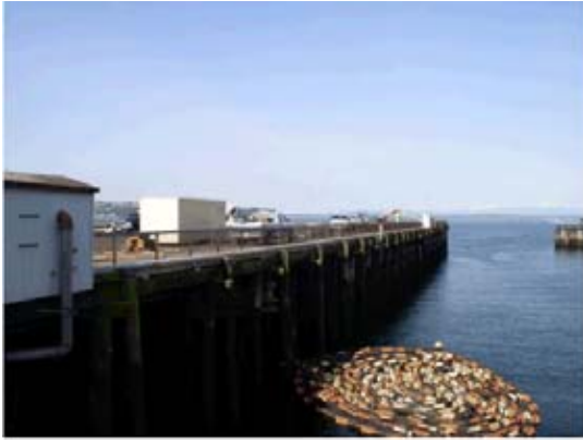
1. View from sidewalk N. Of Pier 62/63 Toward SW
