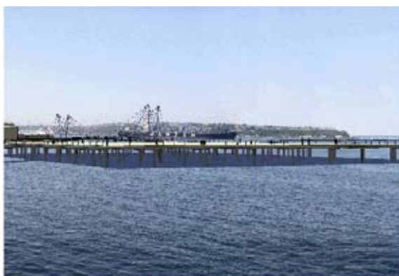
1. View from sidewalk N. Of Pier 62/63 Toward SW
