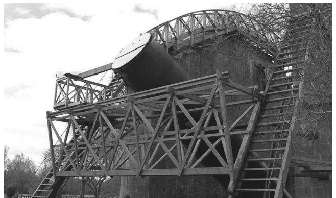
The lower gallery carrying the observing trolley halfway up the track on the inclined 'ladders'. For demonstration purposes only, the telescope and observing platforms are computer controlled.
