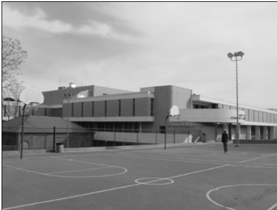
Figure 35. The Marie Reed Community Center, (ca. 1975). Photo taken by KCA Volunteers, 2005.
