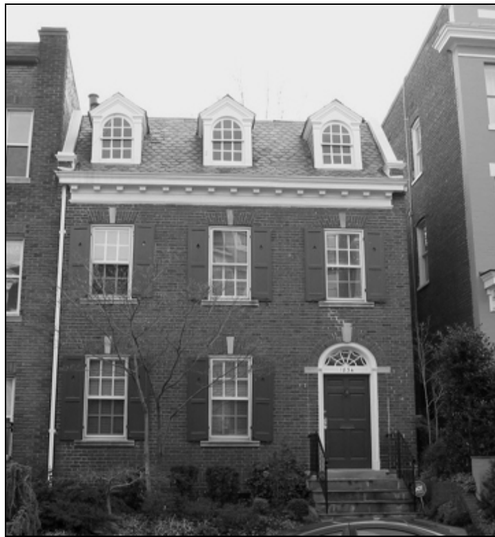
Figure 26. Colonial Revival rowhouse at 1834 Vernon Street, N.W., constructed in 1921. Photo taken by KCA Volunteers, 2005.
