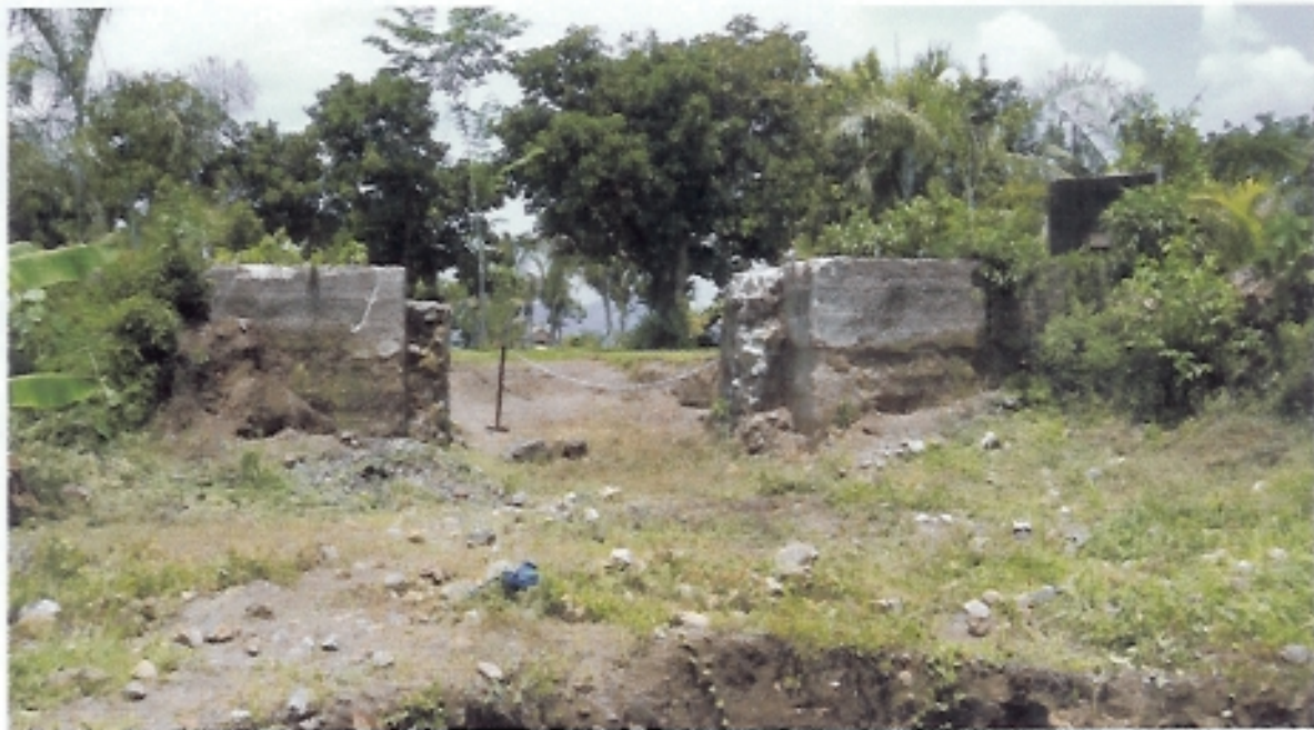
Plate 3. The exposed adobe structures of a ruin.
