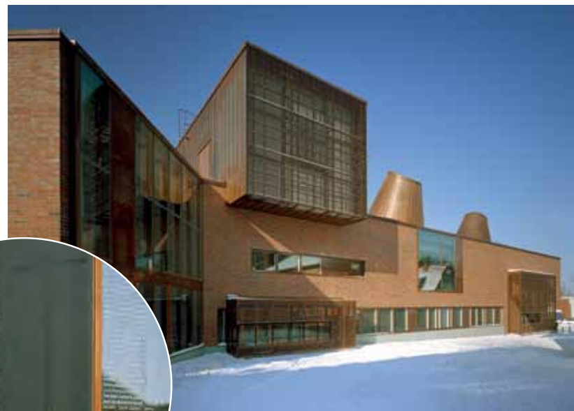
Facade to the east, 2005. The patination of the copper material has begun.
