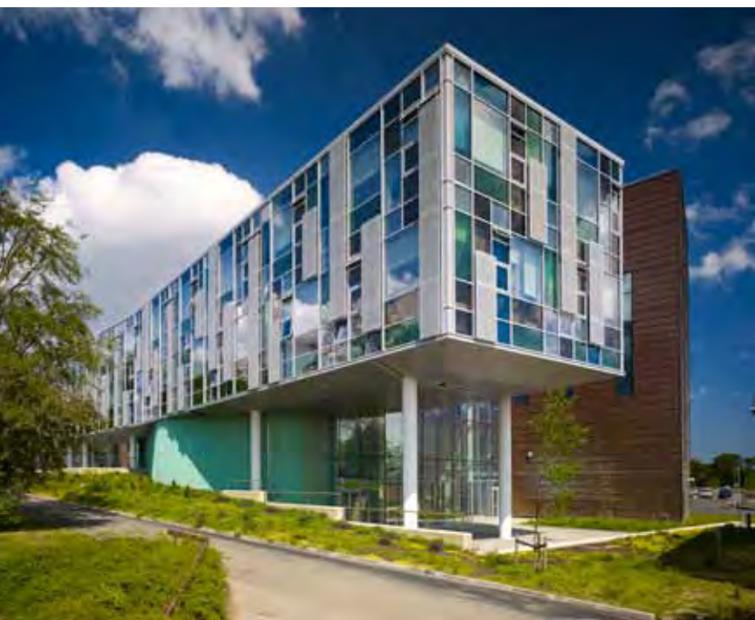
The curved, green pre-patinated copper wall under the glazed wing and brass cladding adjacent reveal two very different manifestations of copper.
