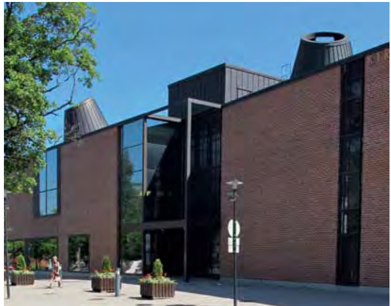
The main entrance of the library, 2011. The copper is fully patinated.
