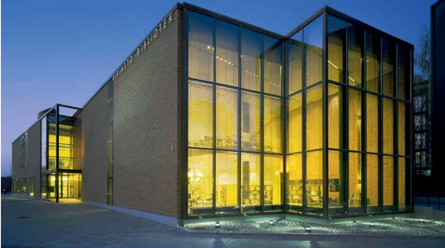
End wall towards the town centre.
