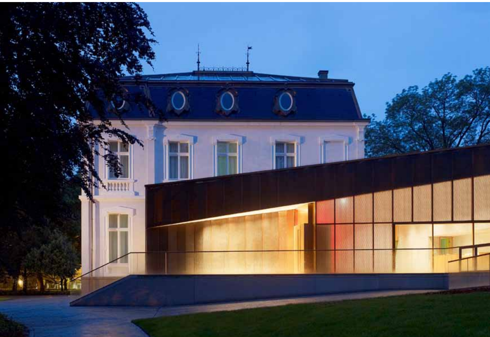
This project was HIGHLY COMMENDED in the 2011 European Copper in Architecture Awards page 14–17.
