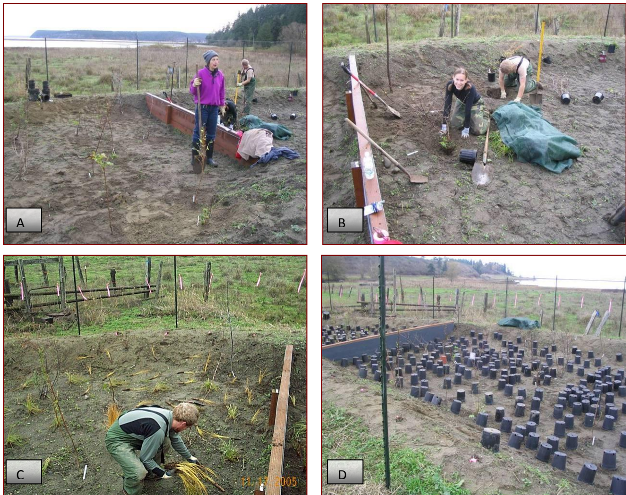
Figure 7. Plants Were Added to the Site in Mirror-Image Distribution in the Two Cells (A-C). After planting, the plant “starts” were covered to protect them from being crushed during mulch application (D).
