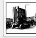
One King West - Installation 9 items
