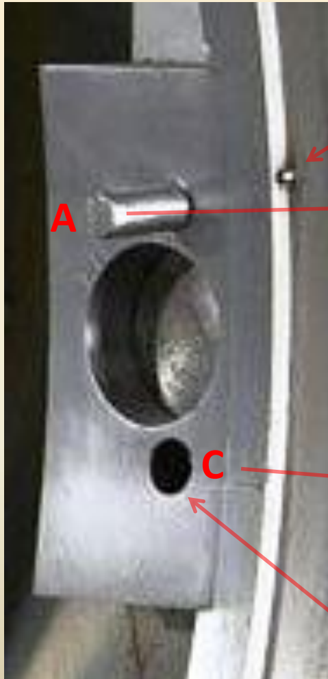
Bolt-Throwing Jamb Pins mounted on interior door jamb
