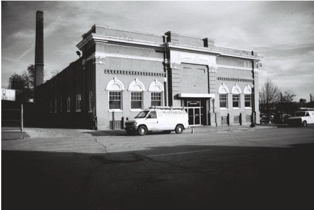
View of the primary (west) and north elevations, looking southeast from across Perry Street.
