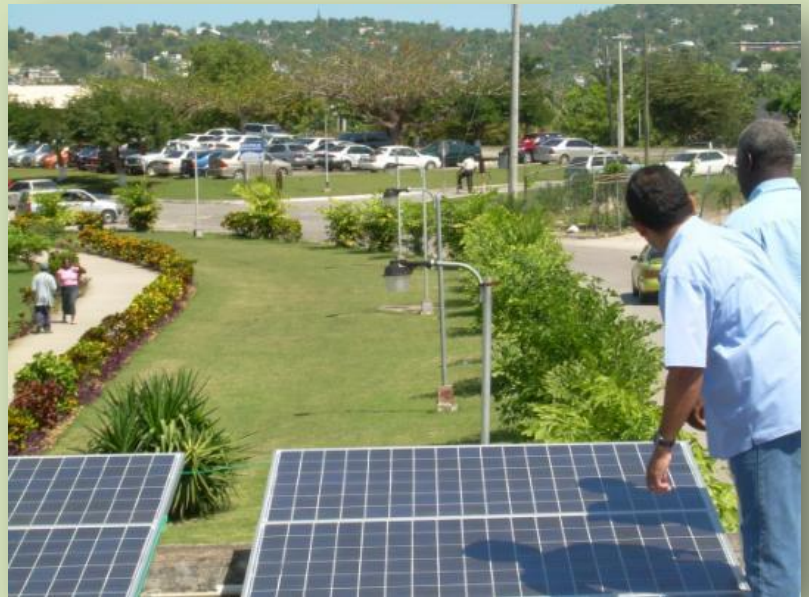
Solar Panels at Cornwall Regional Hospital in Montego Bay
