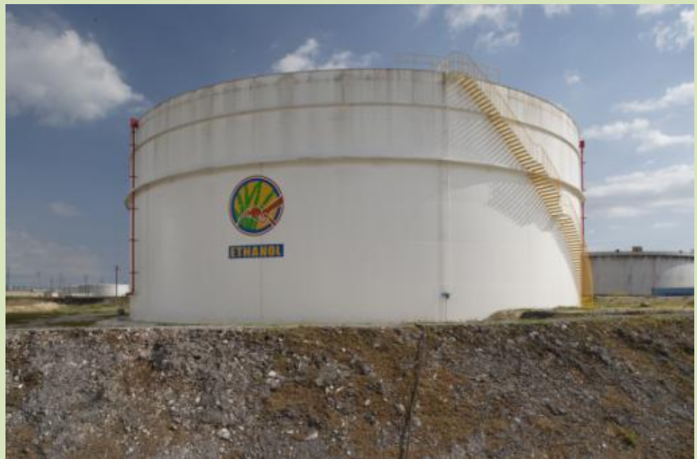
Petrojam Ethanol Storage Tank
