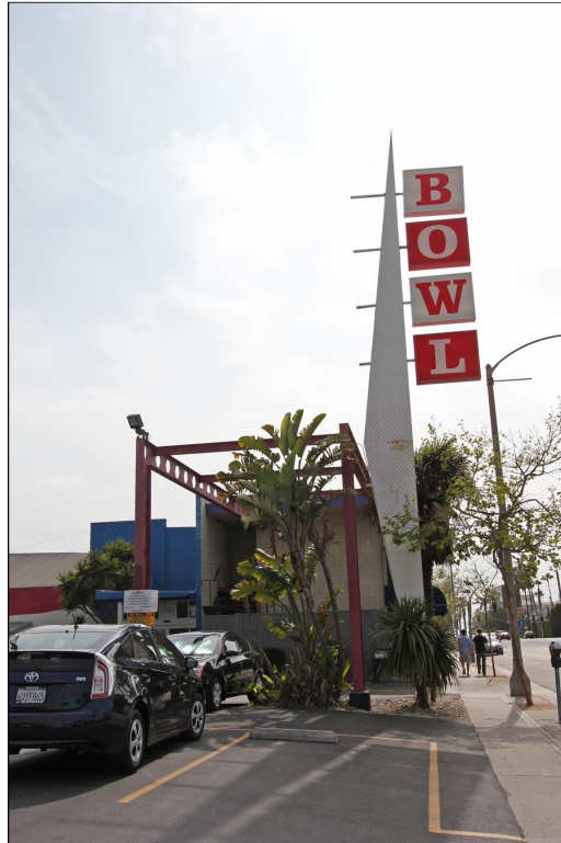
Figure 8: Sign and canopy, view west (Chattel, Inc., 2013)
