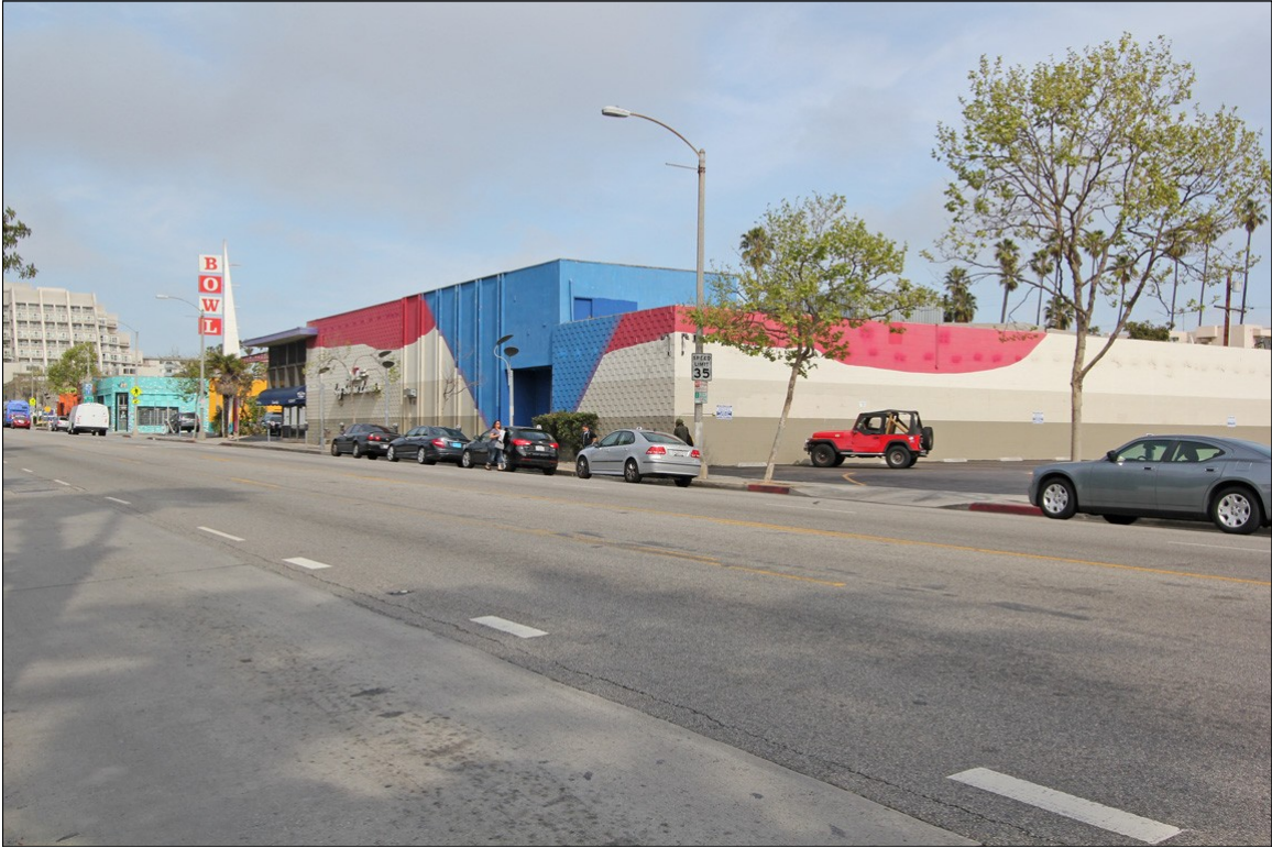
Figure 4: North (left) and west (right) elevations, view southeast along Pico Boulevard (Chattel, Inc., 2013)
