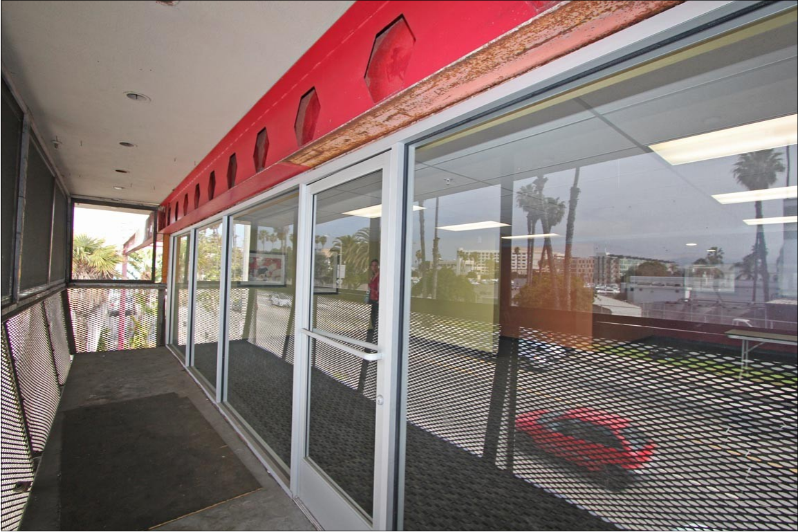
Figure 26: Exterior balcony adjacent to club room, view east (Chattel, Inc., 2013)
