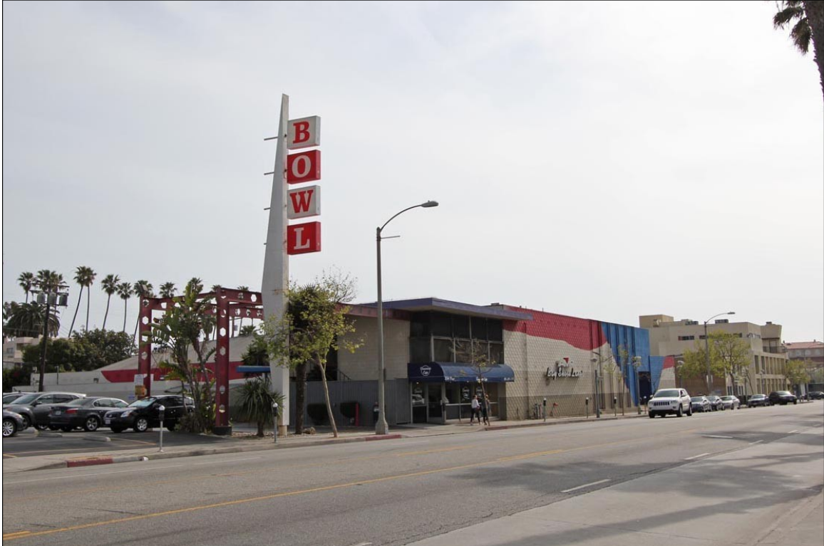
Figure 5: East (left) and north (right) elevations, view southwest along Pico Boulevard (Chattel, Inc., 2013)
