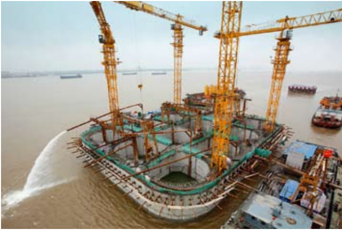
Middle tower foundation under construction.
