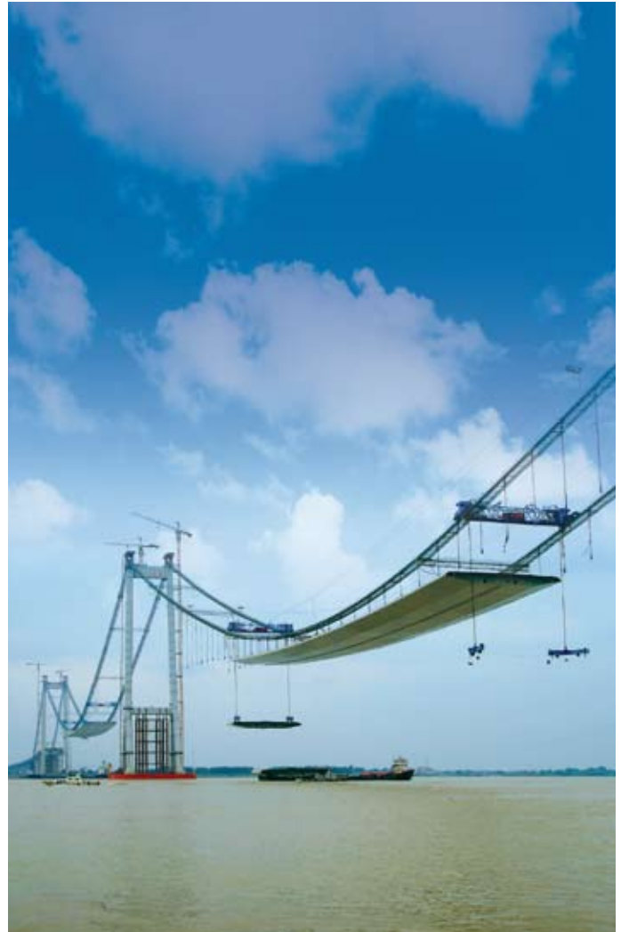
View of the Taizhou Bridge under construction.
