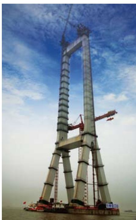
Middle tower under construction.
