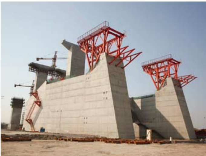
South anchorage under construction.
