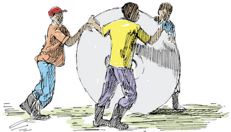
Figure 6. Circular slabs can be rolled into position, making them easier to move over short distances
