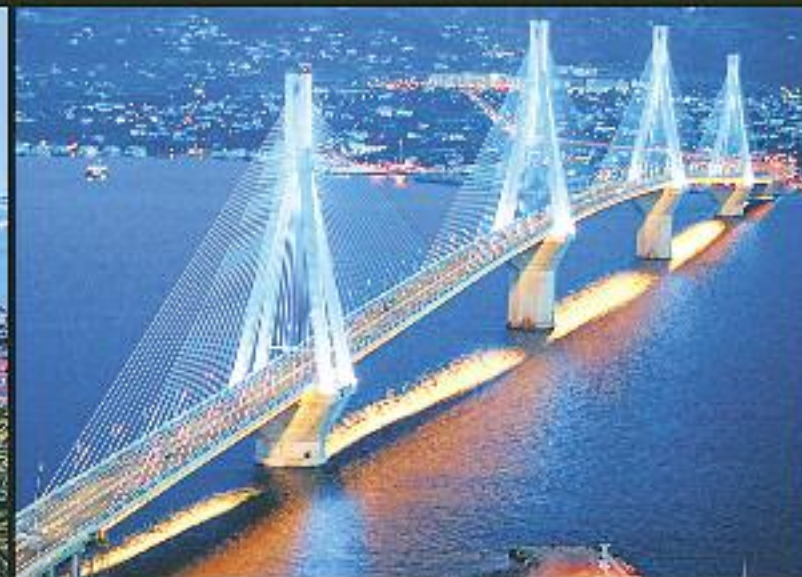
Rion-Antirion Bridge, Corinthian Straits, Patras, Greece
