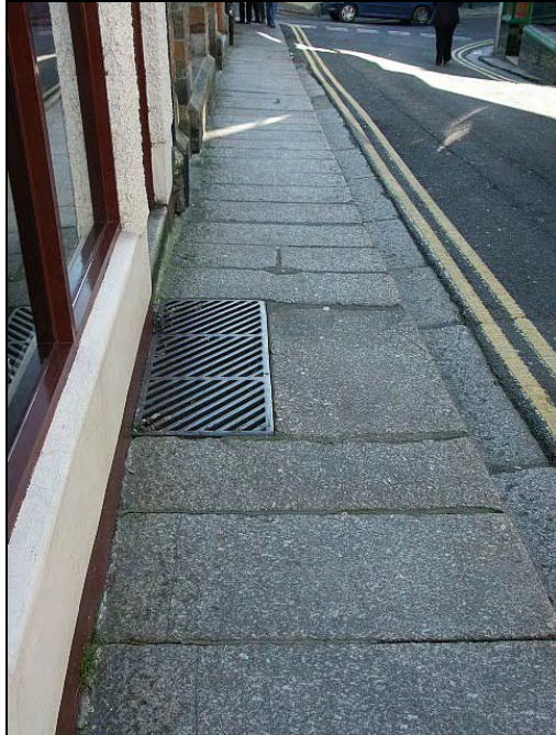
Original granite paving slabs along West Street
