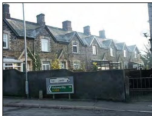
Windsor Cottages, Newport
