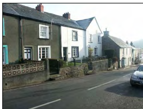
The leat in front of the cottages on St Stephens Hill
