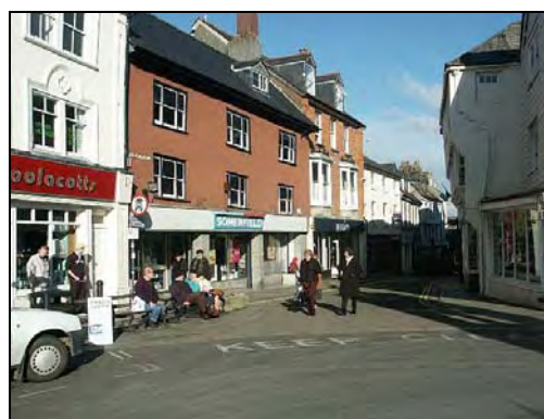
Unsympathetic modern shopfronts in the town centre
