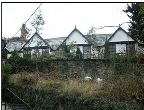
Dockacre House – the east front
