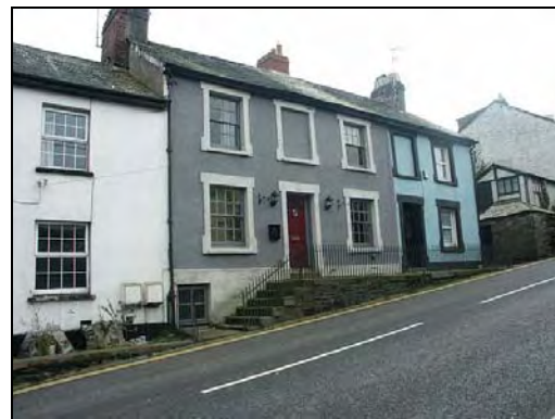
Good quality houses along St Thomas Road under appreciated because of the busy road
