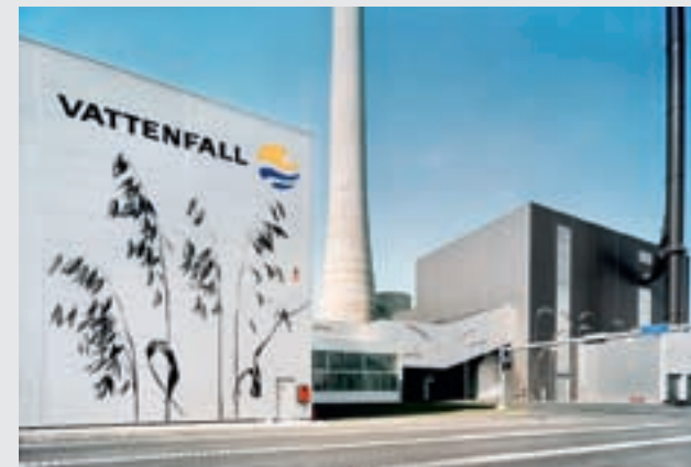
Fyn power station, Denmark.
