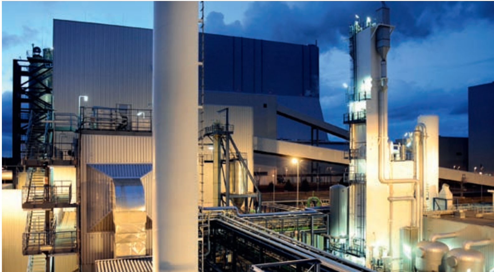
Schwarze Pumpe power plant, Germany.
