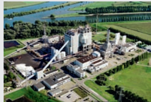
Willem Alexander power station, Buggenum, Netherlands.
