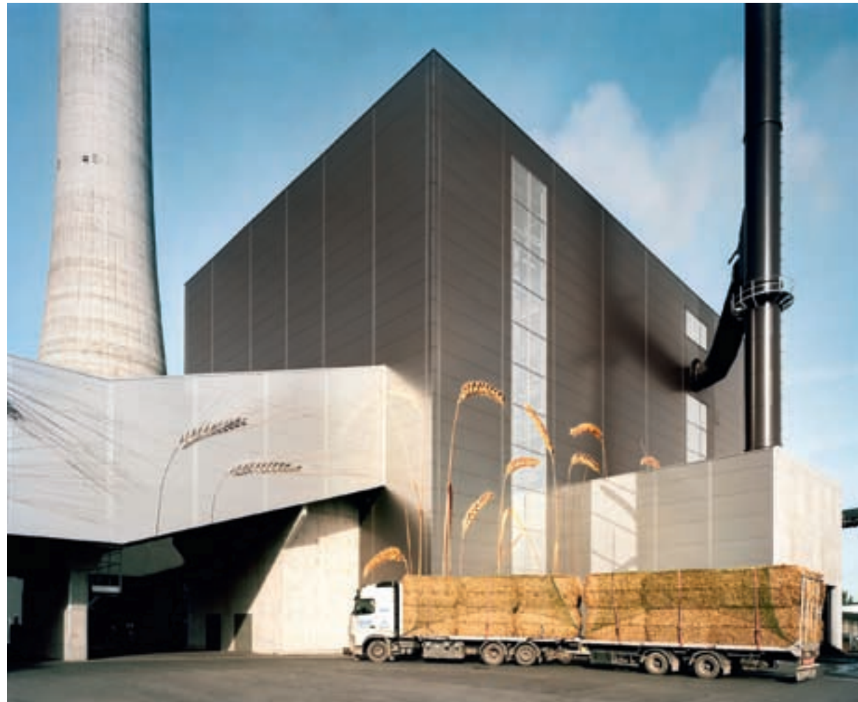
Fyn power station, Denmark.
