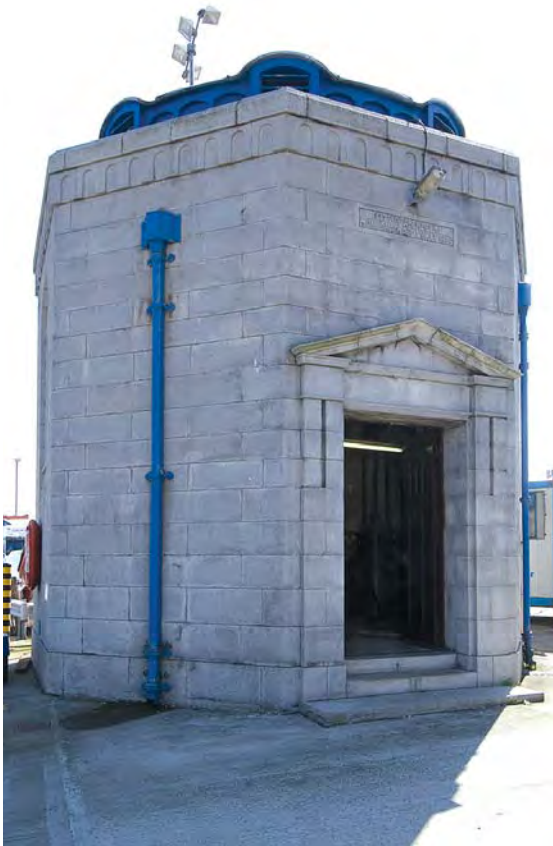
Exterior of Torry Syphon House
