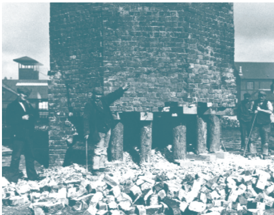
Demolition of the Torry Brickworks chimney in the early 20th century, courtesy of Aberdeen City Libraries
