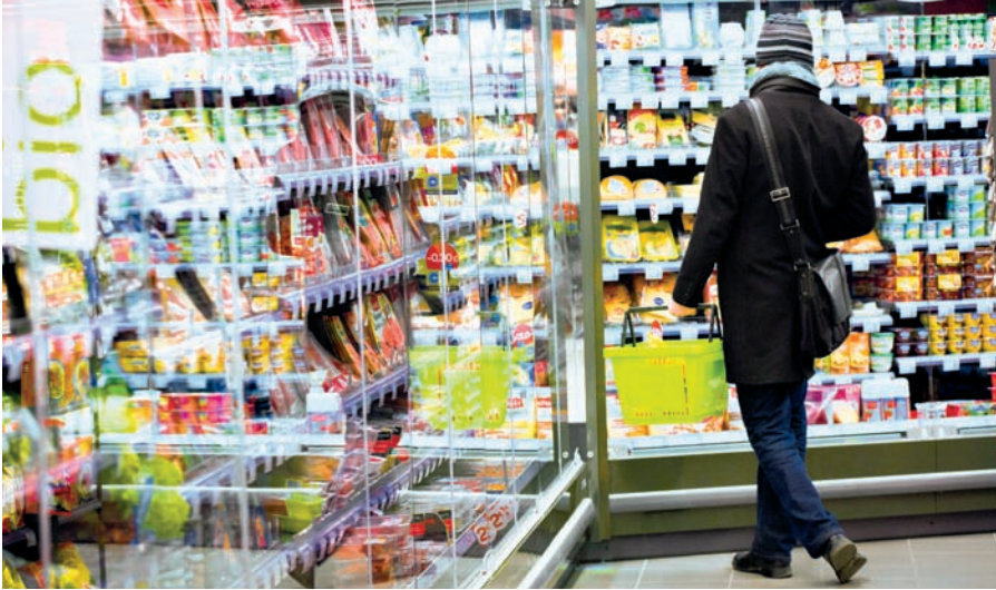
01 Closed refrigeration units is one of the Group's initiatives for reducing energy consumption in its stores. Manhattan Express store in Brussels (Belgium).
