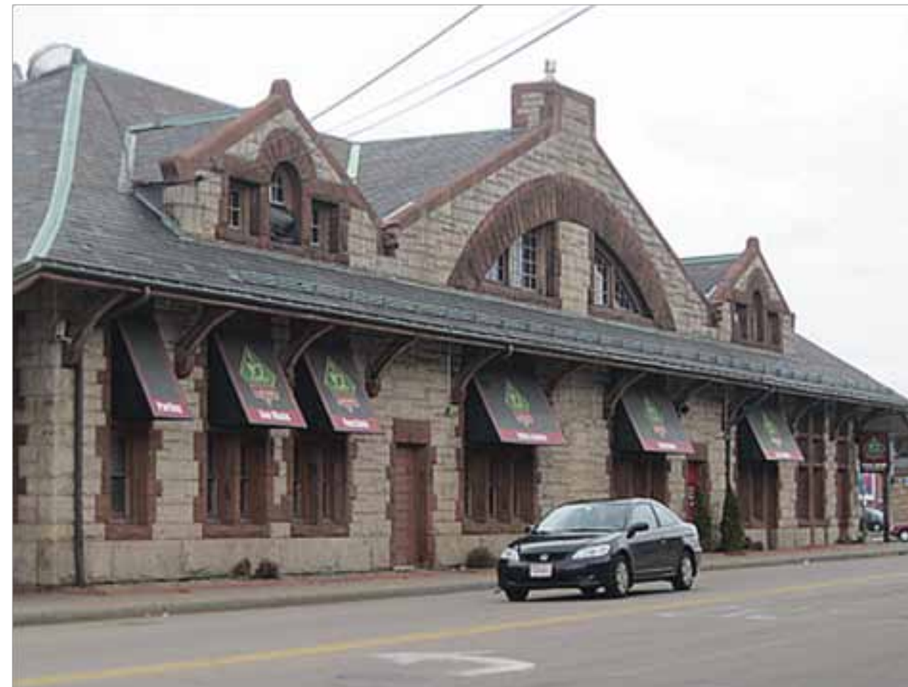
South Framingham Station, 2009
