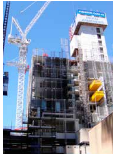
Through close collaboration with engineers, designers and plumbing contractors, Philmac successfully delivered 1,000 Akavents from Akatherm for a new twin tower apartment complex in Sydney (Australia). The ease of installation and reduction in pipework resulted in considerable savings for project developer Meriton.
