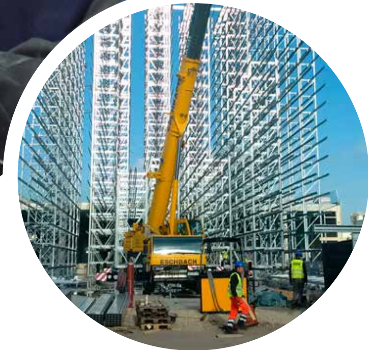
In support of its long-term growth strategy for the electrofusion business, Aliaxis is investing in its logistic capabilities in Mannheim (Germany) with a new, high-bay warehouse, which will allow the group to better serve its customers.
