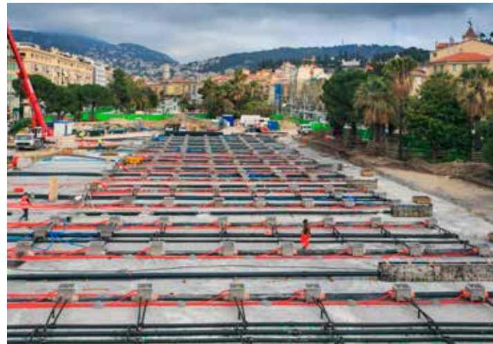
Aliaxis' wide product diversification allowed it to offer the municipality of Nice (France) an end-to-end electrofusion-based solution for a 3,000 m 2 water mirror, part of a major rehabilitation of the city main square. (Picture courtesy of Hervé Fabre Photographie)
