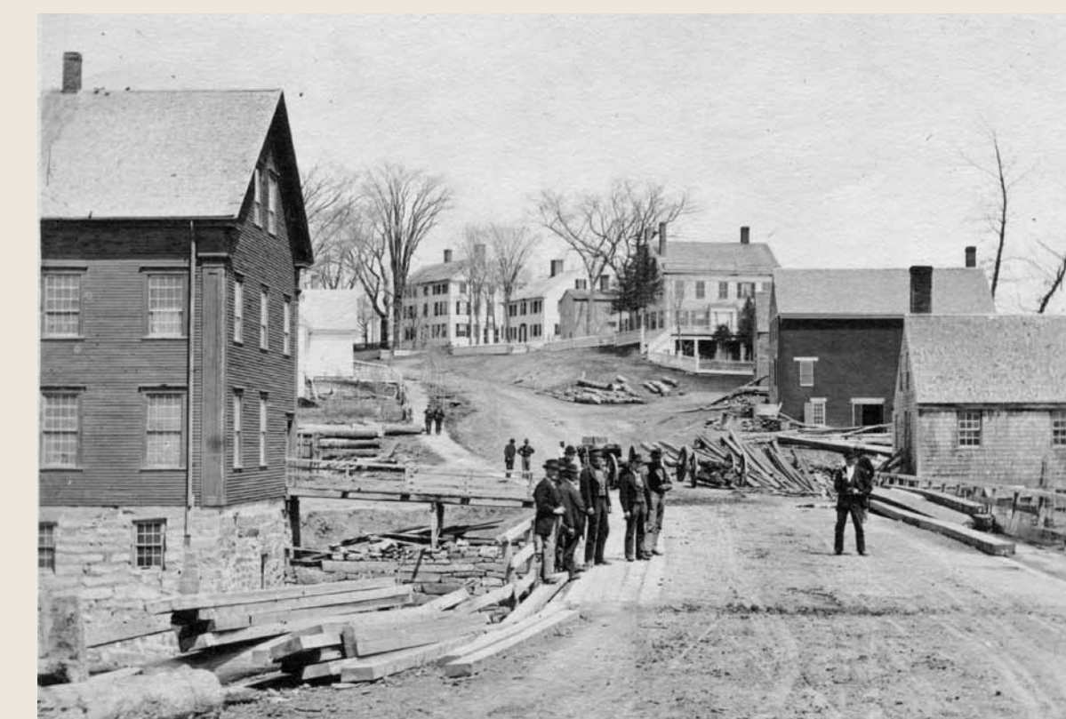
East Main St. hill (Route 88) circa 1874. The foundation of Loring's grist mill on the left supports the overlook in today's Grist Mill Park.
