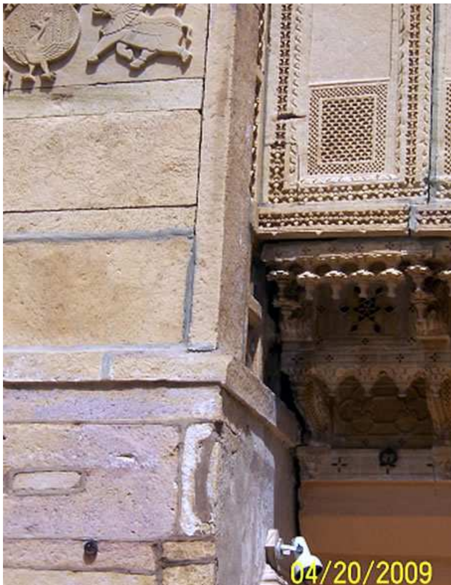
Figure 8: Opening of Joint in Jaisalmer fort
