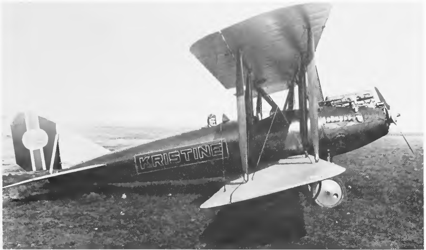
FIGURE 20.—Curtiss Oriole for Amundsen polar expedition, with Curtiss K-6 engine, 1922. (Smithsonian photo A-4602F.)
