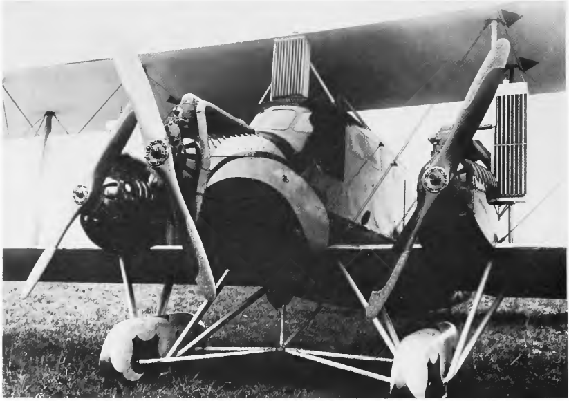
FIGURE 19.—Curtiss Eagle, 1919, powered by three Curtiss K-6 engines. (Smithsonian photo A-4602E.)
