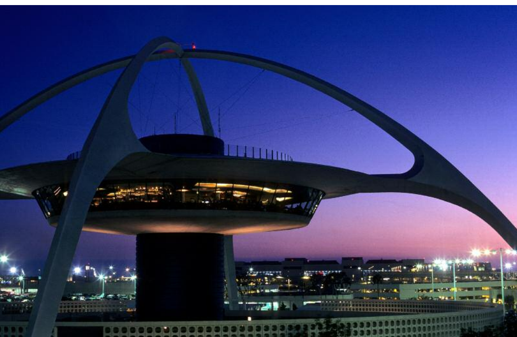
LAX Theme Building, Los Angeles; Photo courtesy Robert Henson
