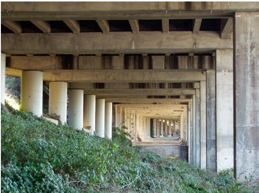
Doyle Drive columns
