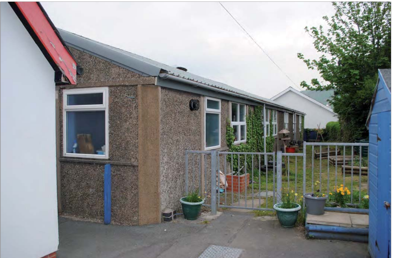
Plate 04: The School Canteen from the South-West
