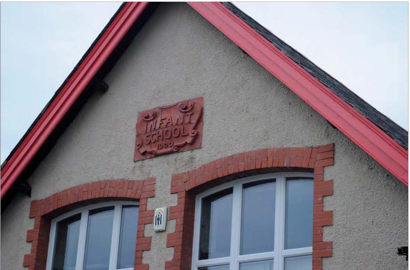
Plate 08: 1900 Terracotta Plaque on Former Infants School Building
