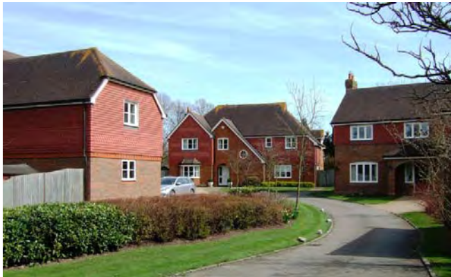
James Close is a recent development of three detached houses on land adjoining James House. Set back from the road around a shared access, the individually designed houses are constructed in red/brown brick with red hung tiles, plain brown tiled roofs and white casement windows. Hedges and protected trees flank the entrance. The development respects the verdant spacious character of this part of the village.
