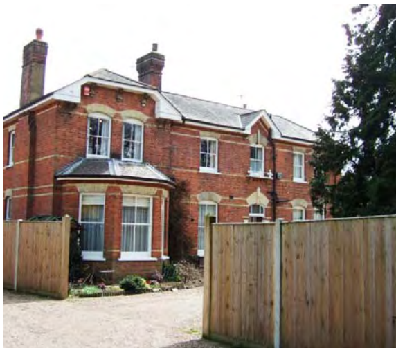
The chapel is part of a small cluster of late Victorian buildings which includes a semi-detached house with prominent white timber details opposite the entrance to Great Elms and the substantial Chesfield which has now been split into two properties. Three detached houses have been constructed in the grounds of Chesfield which replicate the design details of the main house. Two 1970s bungalows occupy land to the north set back from the road down a private access.
