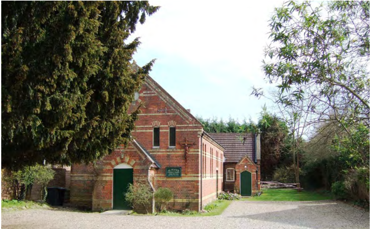
St Peter's Catholic chapel is set back from the road behind a deep gravel unenclosed parking area which creates a gap in the road frontage. Conifers frame the building to the rear. Formerly a Gospel Hall, the building was constructed in the late 19 th century and has distinctive contrast yellow brick bands and decorative arches over windows and doors. Southwards from this point evolving vistas open up of key landmarks of the Conservation Area - Hadlow Castle Tower and surrounding Wellingtonia trees and St Mary's Church Tower.
