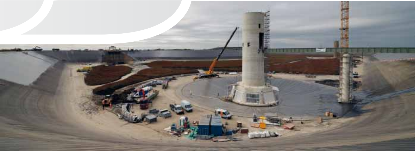
STRABAG - Construction site of pumped storage hydropower plant, Vianden, Luxemburg
