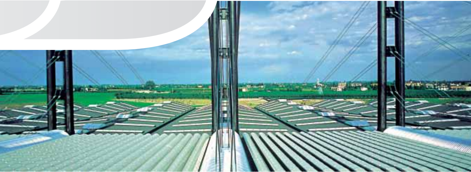
BENETTON – Castrette industrial complex, Villorba, Treviso, Italy
