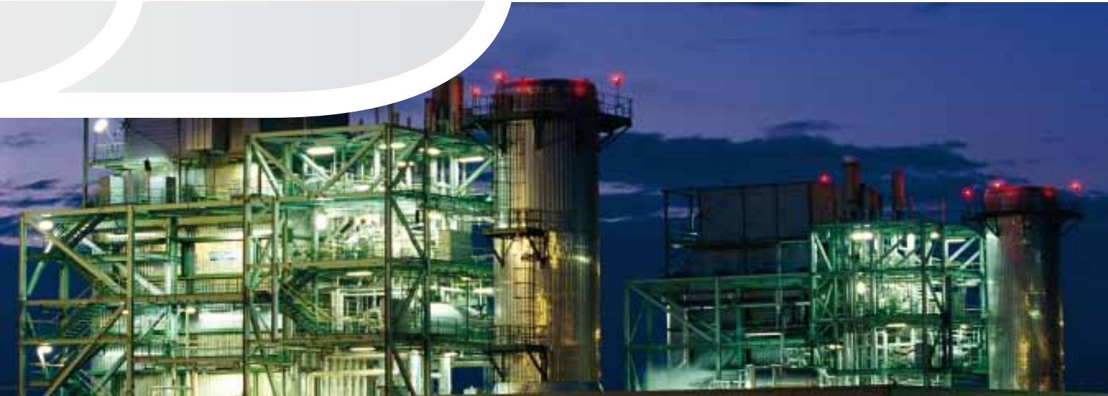
ACEA - Tor di Valle thermoelectric power station, Rome, Italy
