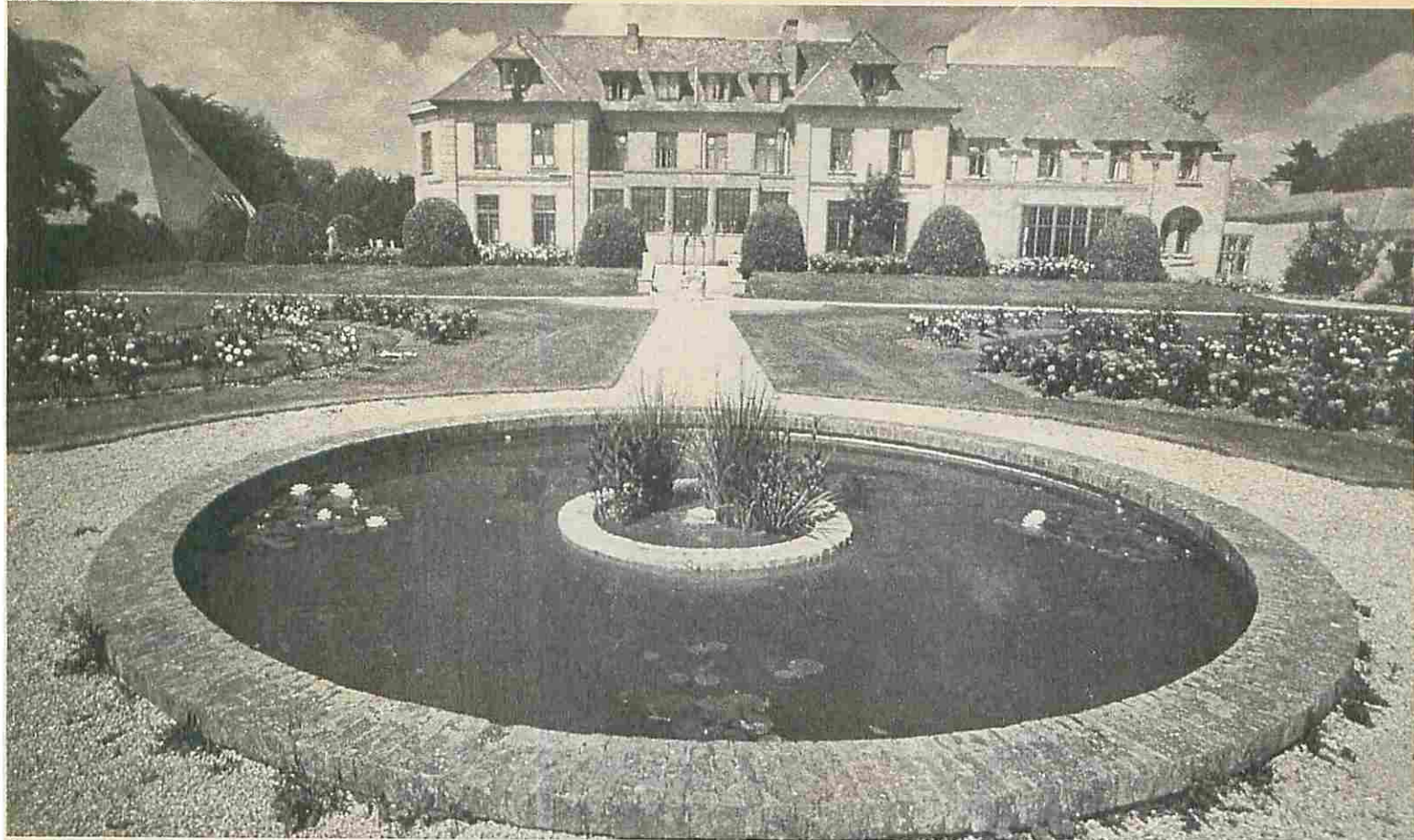
View from the sunken garden of the back of the college, with Sir Basil Spence's pyramid-shaped building, designed as a concert hall and now empty, on the left.
