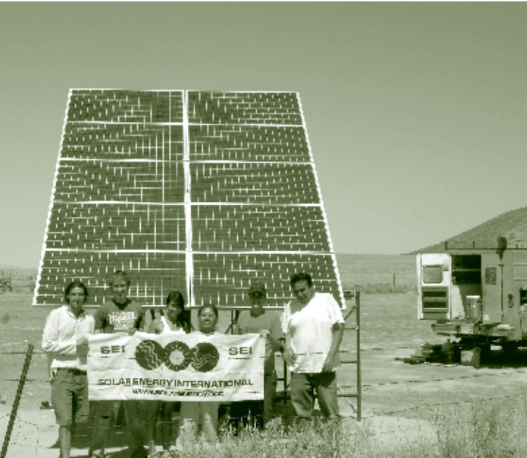
Honor the Earth and Solar Energy International install a solar panel on the Skull Valley Goshute Reservation. Photo: Honor the Earth.
