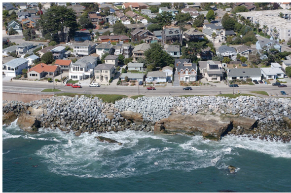
West Cliff Drive seawalls Santa Cruz 2004
