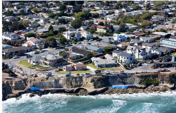
Pleasure Point Seawall under construction 2004 (denied by CCC Nov. '03)
