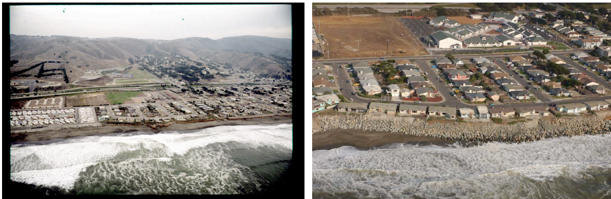
Shoreview seawall Pacifica: before (c. 1979) and after (2004)
