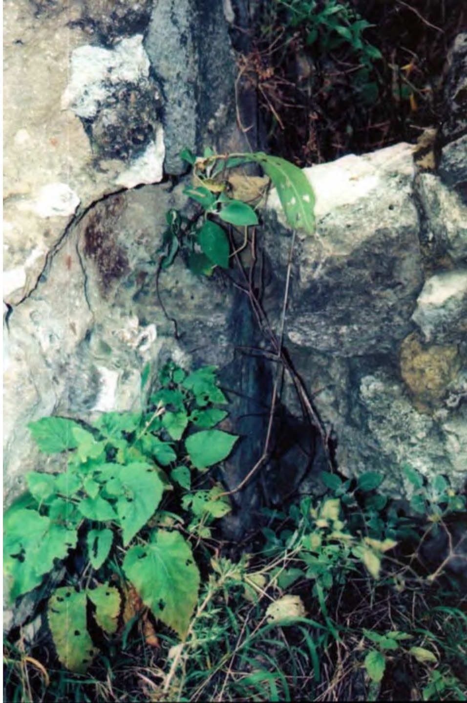
Figure 19. Structure 4 Wall Truncated by Church.
