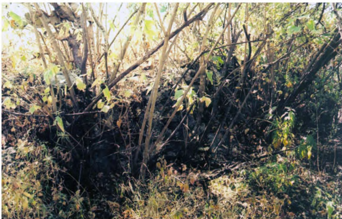
Figure 24. Platform 10 West Retaining Wall (Facing Stone).
