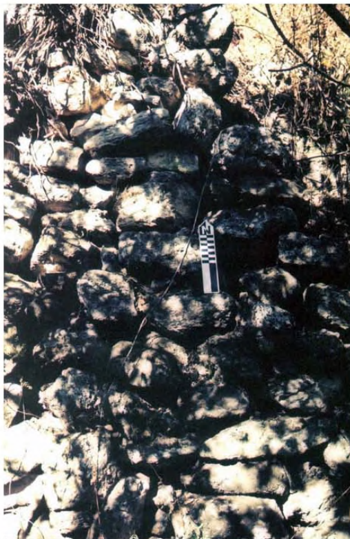
East Retaining Wall (Rubble Core and Facing Stones)
