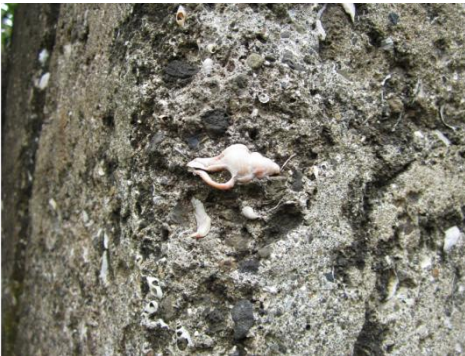
Plate 16. Chicoreus capucinus as part of the wall construction.
