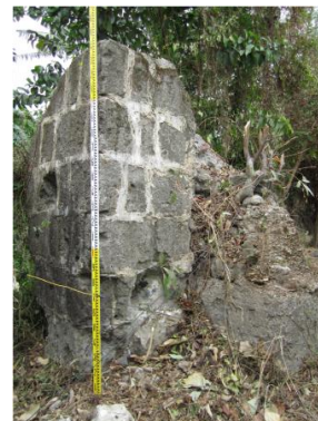
Plate 6. Documentation of masonry structures
