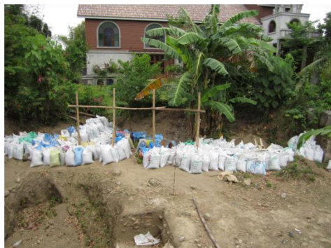
Plate 8. Backfilling the site
