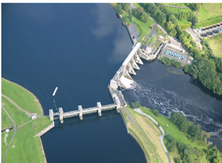
Parteen regulating weir on the Lower River Shannon, showing the weir structure which diverts water through the headrace canal to Ardnacrusha hydroelectric station. The location of the Parteen hatchery unit, where some of the experimental rearing of salmon will take place, is also shown.
