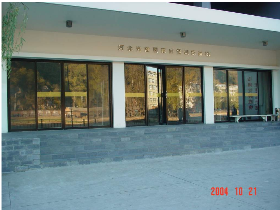
Comprehensive building in Hebei Xinglong National Athletic Training Base (for administration, reception, etc.)
