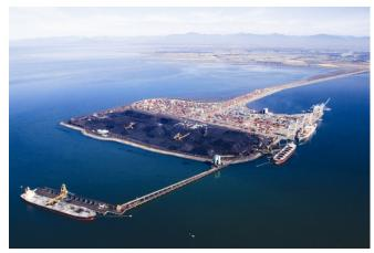
The Westshore Terminals operation at Roberts Bank near Vancouver currently ships around 25 million tonnes of coal per year and has recently expanded to increased capacity. The province has deep water ports near Vancouver, mid-coast at Prince Rupert and toward the north at Stewart.
