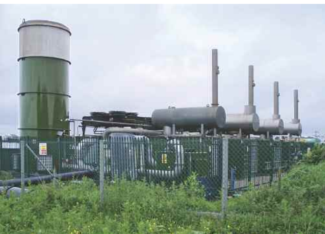
These four power plants at the Cathkin landfill outside Glasgow generate about 30,000 MWh annually from captured methane.
