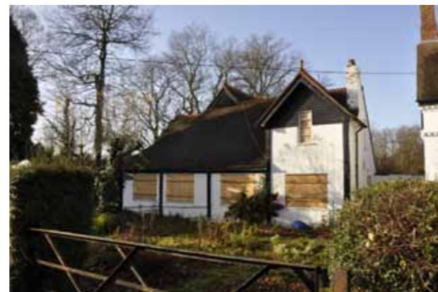
Ancillary building, potentially former School Master's house
