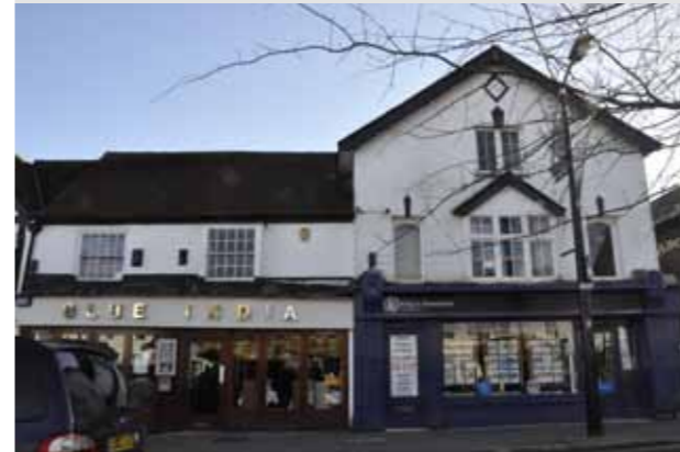
No. 47a High Street on the left and No. 45 is on the right
