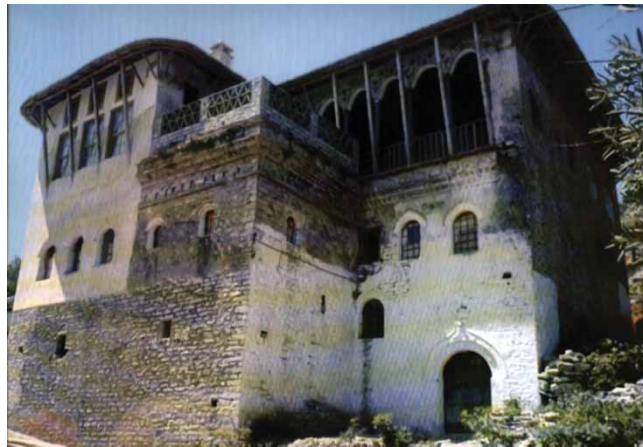
Figure 16. Kamerie topped by a veranda. Photo courtesy of the Institute of Cultural Monuments.
