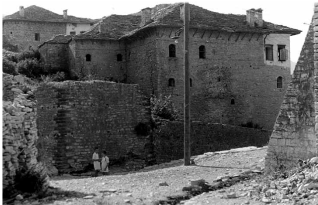
Figure 14. Side and back façades with minimal openings. Photo by Branimir Gušić c. 1947.
