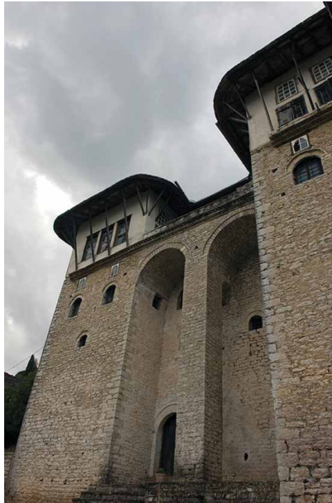
Figure 9. Zekate residence, one of Gjirokastra's most monumental houses. Photo courtesy of Cultural Heritage without Borders, Albania.
