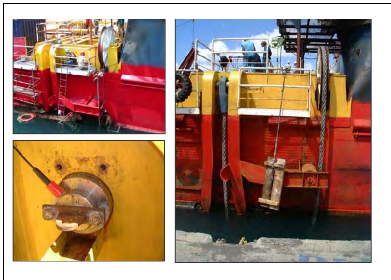
Figure 5-17. ROCKWATER 2 Prepared for Lifting (Top left, the lifting sheave has been installed. Bottom left, the load cell measures the tension on the end of the lift wire. Right, the lift wire is installed for testing.)
