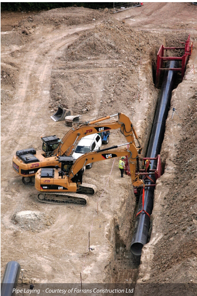
Pipeline working strip - Courtesy of Farrans Construction Ltd
