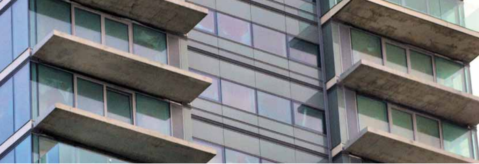
Concrete balconies thermally separated by Schöck Isokorb® K
