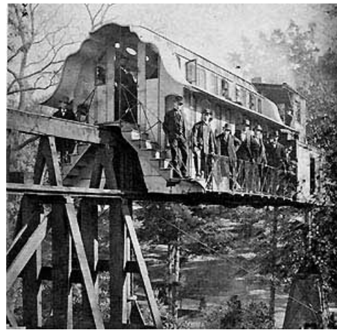
General LeRoy Stone's steam engine monorail
