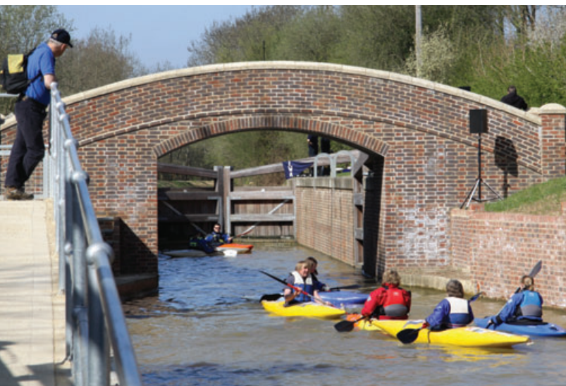
Loxwood Lock and horse bridge - the new parapets will be built with similar materials
