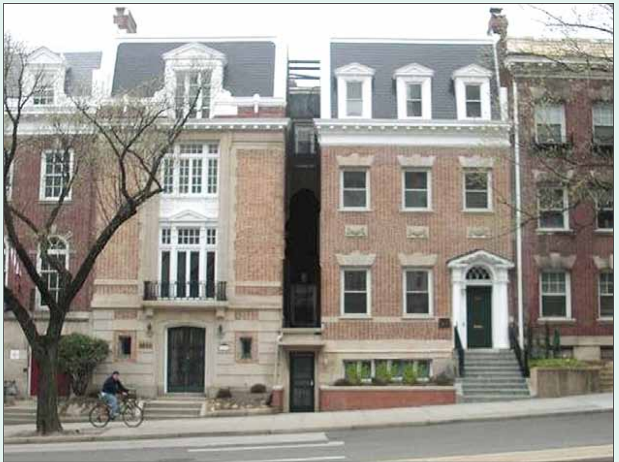
2010 view of 1832 (left) and 1834 (right) Connecticut Avenue, NW.
