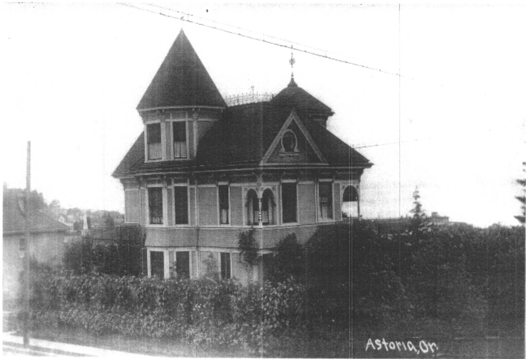
The Judge Charles Page-Samuel Elmore residence was converted to apartments After Astoria's downtown burned in 1922. Fig. 21
