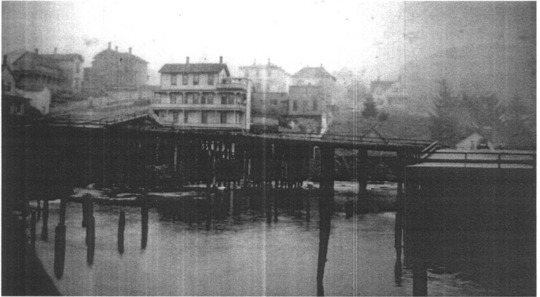
One block below the Shively-McClure District, streets were constructed on wood pilings above the river. The residential neighborhood was constructed above the river bank. Looking south, one block below Franklin Avenue between 13th and 14th streets. (photo courtesy of Clatsop County Historical Society)
