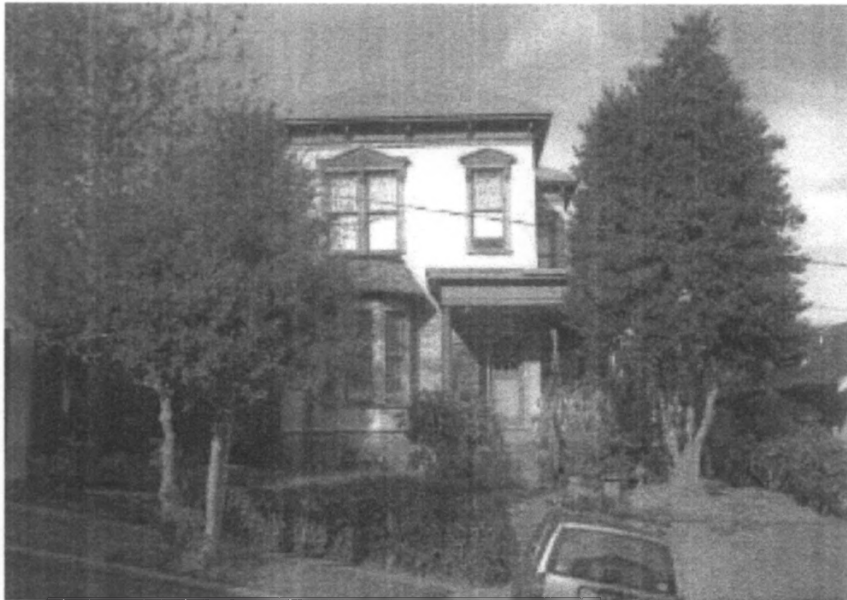
B). M.D. Kant residence constructed in 1880. Fig. 15
